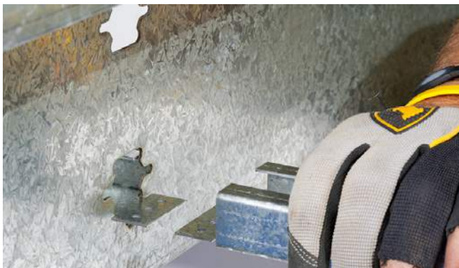
Purlin Keyway - simple roofing screw assembly
