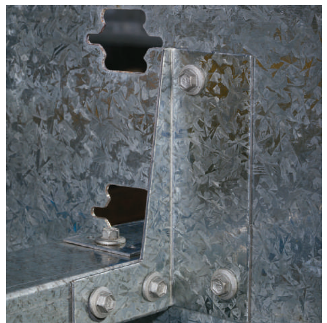
Bridge Bar Stabiliser - prevents purlin 'roll'
